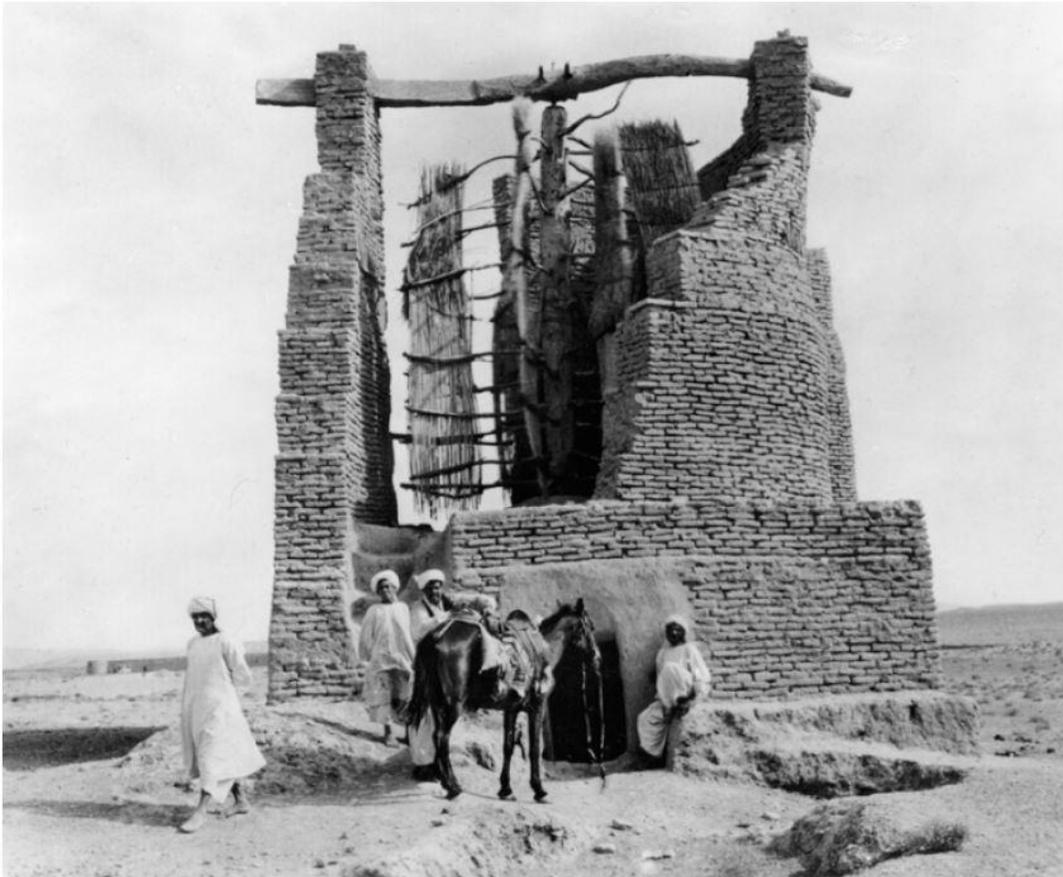
*Figure 5 VAWT for milling grains [1]*
