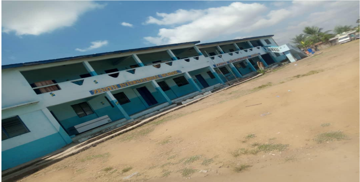
7. A picture of the Building structure of one of the private schools in the research area
