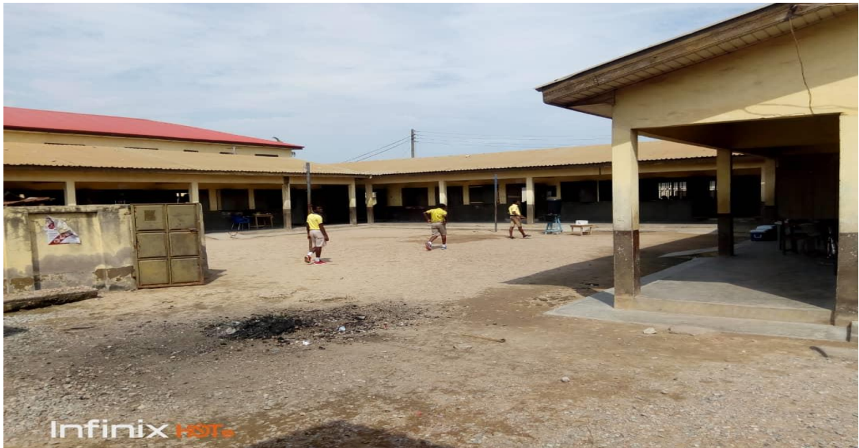
8. A picture of the Building Structure of a Public school in the research area
