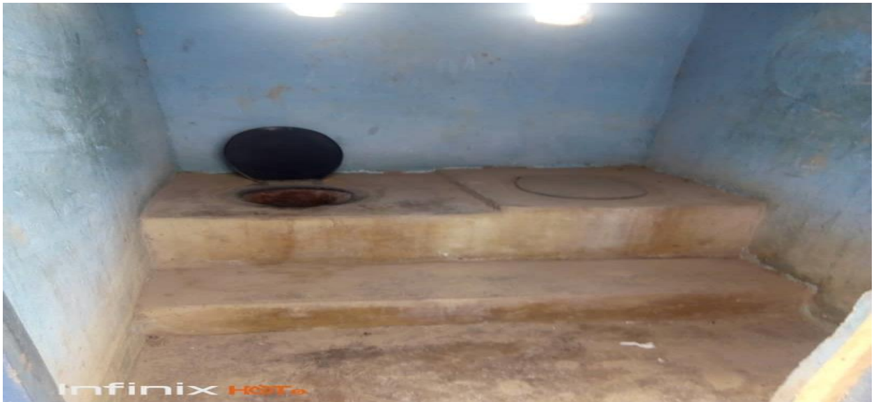
6. A picture of Public schools toilet facility from the research area
