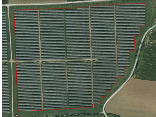
Figure 3-13 Solar Park RICH satellite picture [38]
