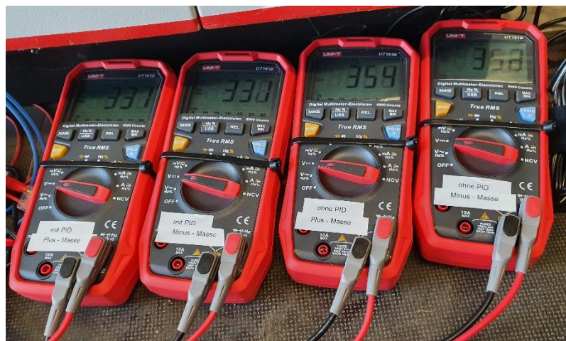
Figure 3-28 Installation of the dedicated voltage measurement
