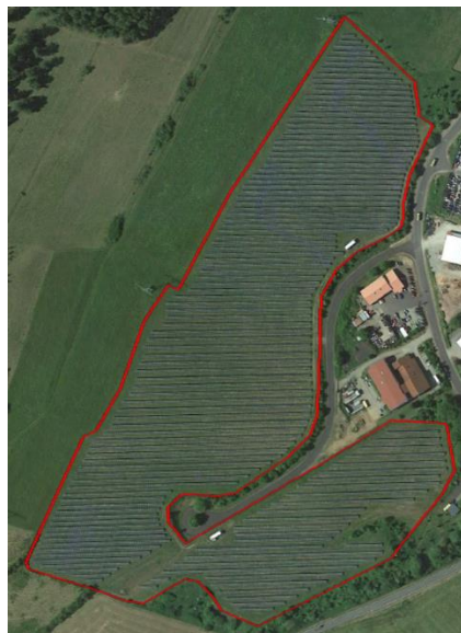
Figure 3-24 Solar Park Thuringia South satellite picture [38]
