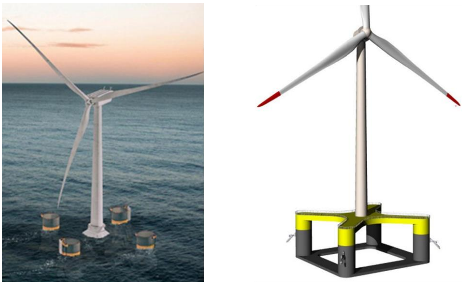
Figure 15: Square semi-submersibles (from left to right): XCF from Marel, Nautilus from Nautilus Floating Solutions [57], [58]
