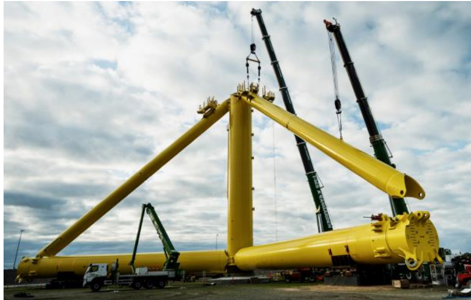
Figure 25: Substructure assembly of TetraSpar from Stiesdal [41]
