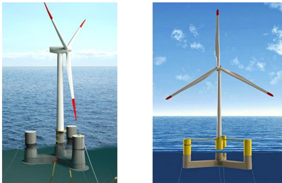
Figure 12: Concrete semi-submersibles (from left to right): OO-Star from Olav Olsen, VoltturnUS from UMaine [48], [49]
