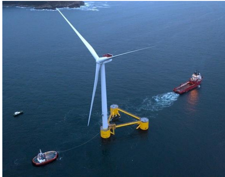
Figure 34: Towing operation of the WindFloat from Principle Power [99]
