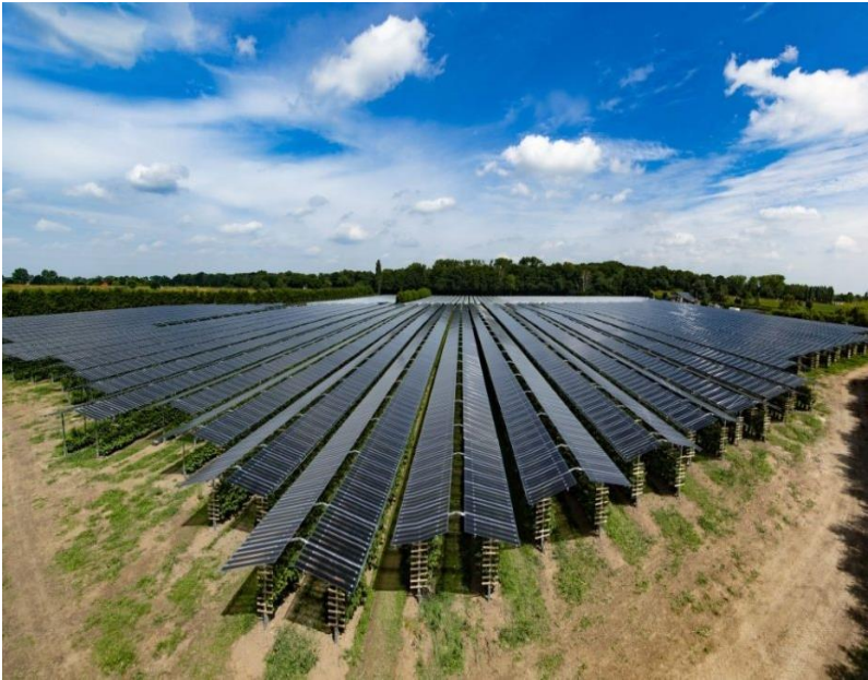
Figure 6: Overhead static system over berries in Netherland © BayWa r.e. and GroenLeven
