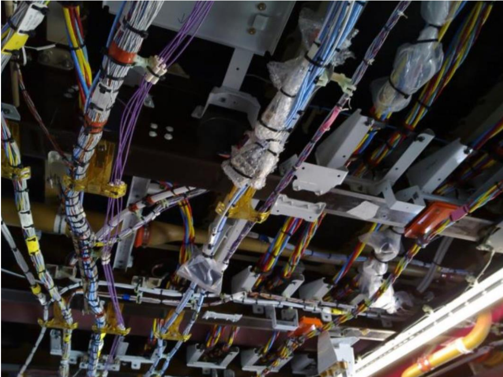
Figure 3.11 Typical wiring installation in A380 crown area (AVSI 2015)
