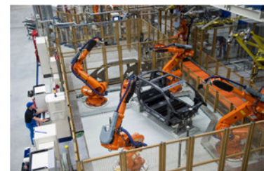
Figure 1.1: Caged safety zone around multiple robotic arms in an industrial environment
