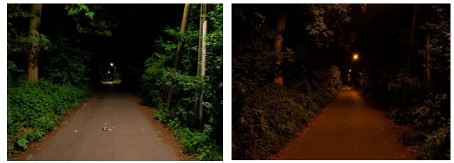
FIG. 1 PILOT PROJECT 'BULLNWSCH'; LEFT: OLD INSTALLATION BEFORE MODIFICATION, WARM WHITE AT 3000 K LIGHT BUT LOW UNIFORMITY AT STREET LEVEL; RIGHT: NEW INSTALLATION AFTER MODIFICATION WITH WARMER COLOURED LIGHT AT 2200 K AND HIGH UNIFORMITY AT STREET LEVEL (PHOTOS: C. LIEDTKE)
