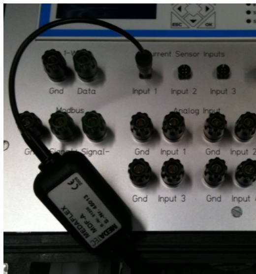
Figure 9.10.: Installation of a Medaflex clamp-on ammeter
