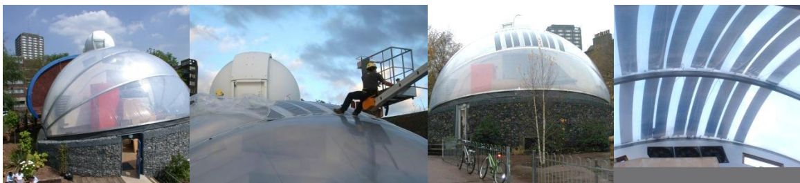
Abb. 49: ETFE-Kuppel des Classroom of the Future London, 2006 [ http://www.vector-foiltec.com/cms/de/projects/type/typelistcs.php?recordID=21 ]
