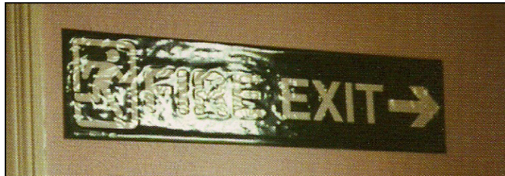
Figure 40: Glare caused by the shiny surface of the sign [13]
