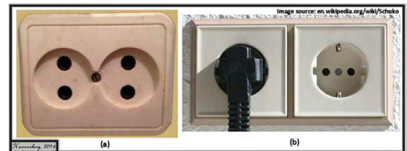
Figure 17: Electric sockets in Mongolia (a) and in most of Europe (b). Electric frequency and Voltage is the same, the European plugs can be connected with the Mongolian sockets, but with a number of disadvantages.
