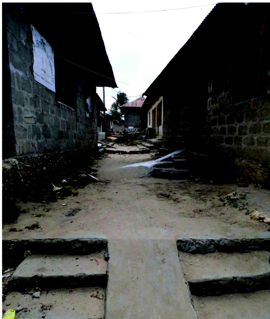
Steps with ramp
