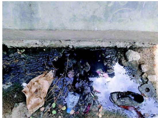
Stagnant water from domestic outflow
