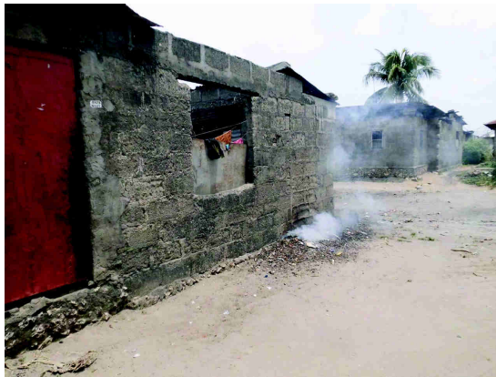
Burning waste next to house
