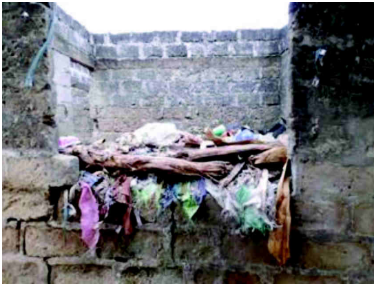
Waste disposal abandoned house - Nyerere
