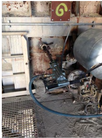
Figure 17: Drill machine and big blaster
