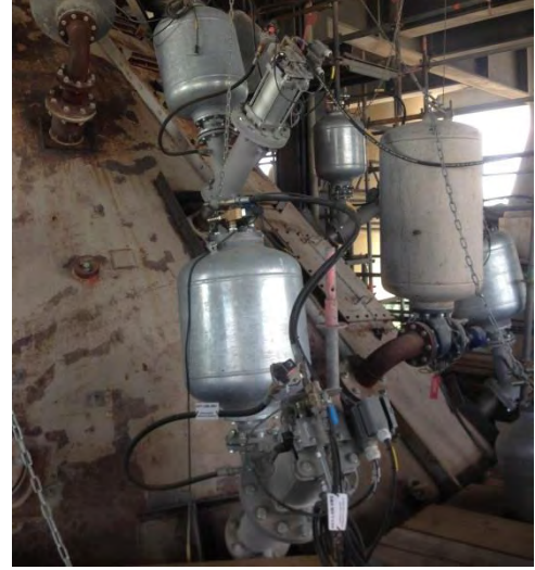
Figure 22: Big blasters at the calciner
