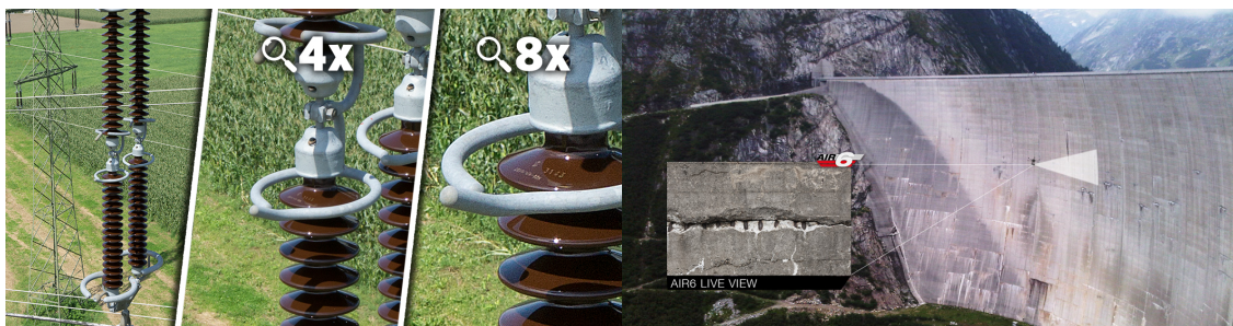
Figure 3: Magnified pictures of a transmission line and a barrage inspection by using a UAV.
