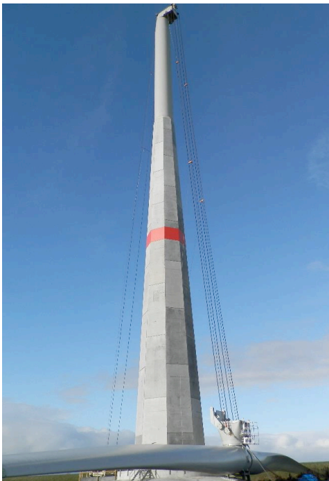
(2) SkyWind SW 3.4 MW during installation via the integrated winch system at Husum
