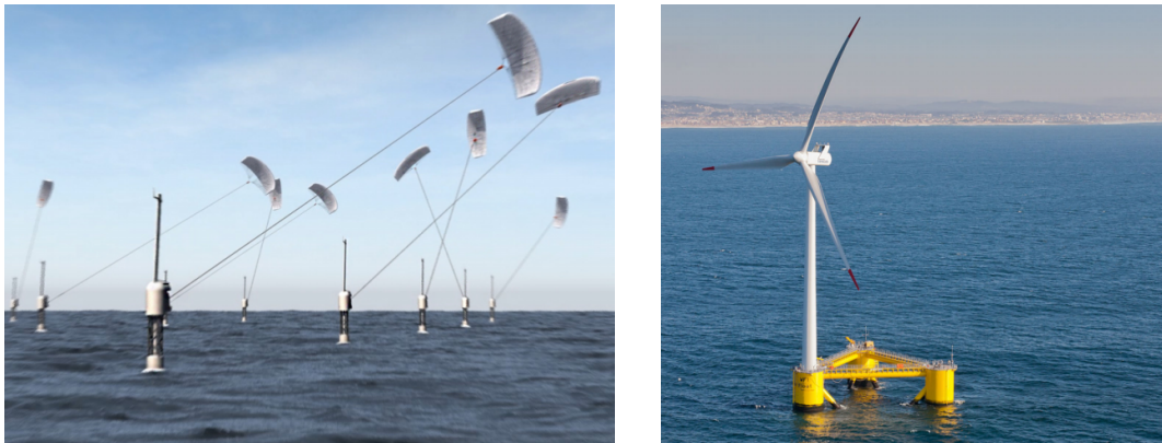
Figure 2-2: Offshore airborne wind energy system (left) (EnBW 2018e) and a floating offshore WTG off the Portuguese coast (right) (EnBW 2017b)
