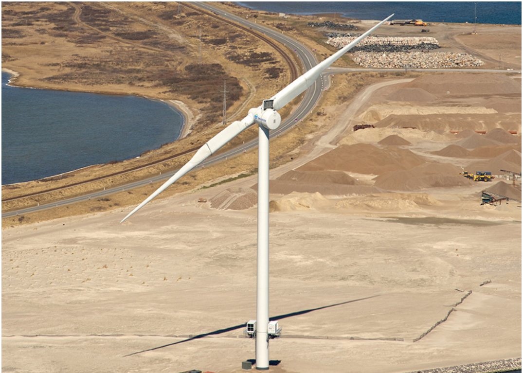
(1) Envision EN-128/3.6 PP 2B (or GC1) 3.6 MW at Thyborøn test field in Denmark
