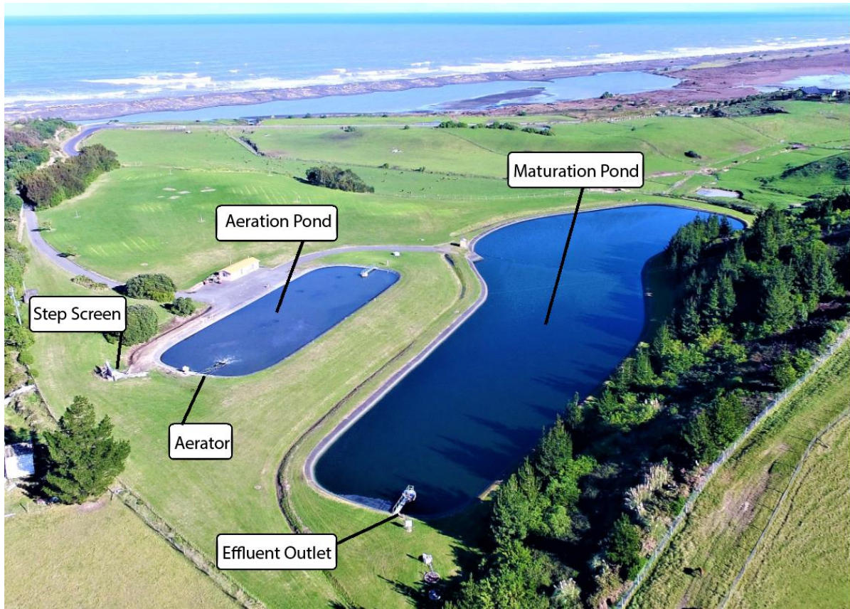
Figure 3-1 Structure of Wairoa Treatment Plant (own image recording)
