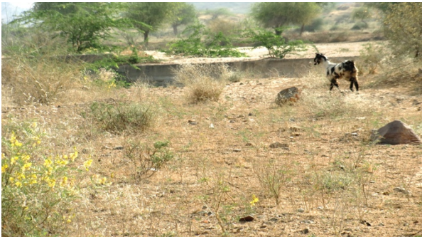
Figure 13: Cattle crossing over the sand dam. Image taken by author 22.03.2017.
