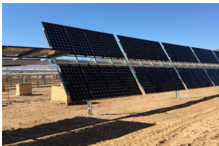
Figure 3.14.a) Power plant of 1.7 MW with single axis tracking in La Silla, Chile and b) portrait configuration of trackers with bifacial modules [Biz17]
