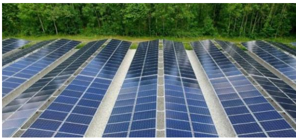
Figure 3.13.a) Horizontal East-West oriented 400 kWp (front side only) bifacial PV plant b) System design parameters for the power plant [Ver17].
