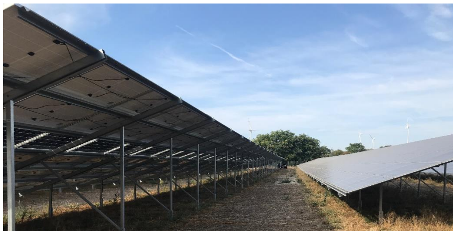
Figure 6.2. Photograph showing part of the setup of monofacial and bifacial modules installed at Dornstedt in Germany (Enerparc AG)
