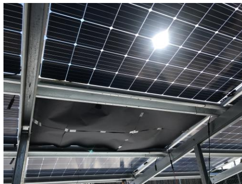
Figure 6.14. Experimental set-up for the measurements of the power output of just the front side of the bifacial module.
